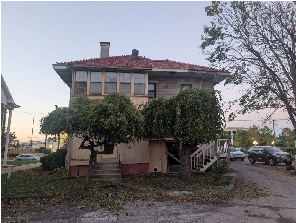
Photo 5 – Back Side Elevation; Facing North
