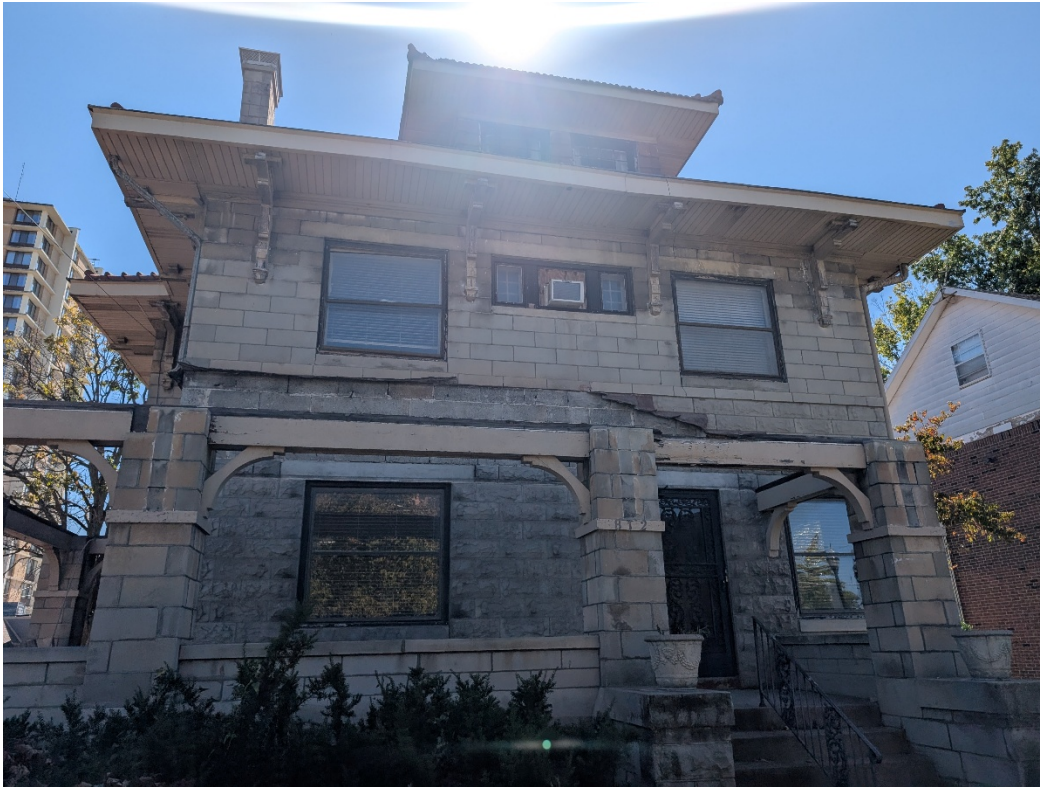
Photo 1 – Front Elevation; Facing South
