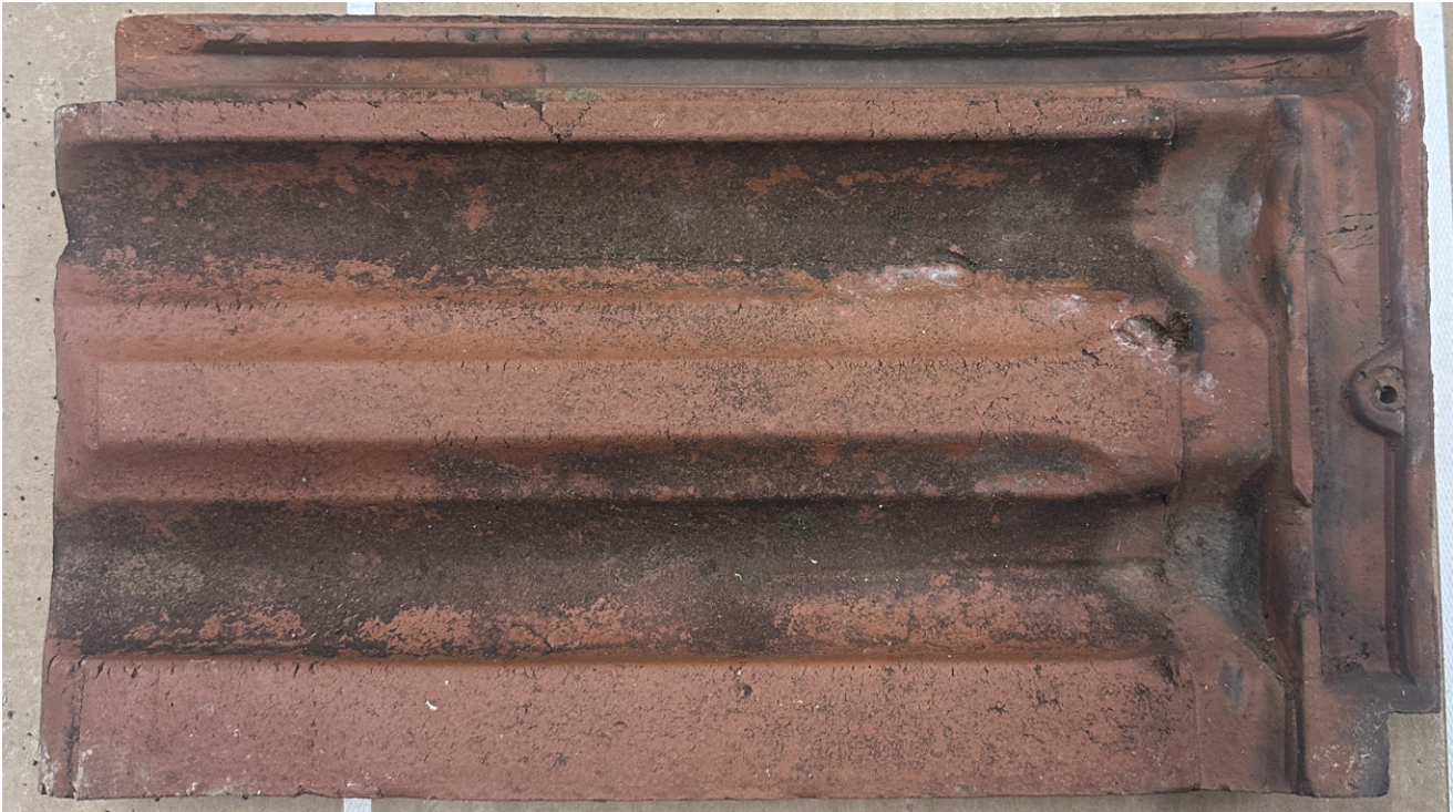
UNDERSIDE OF SHINGLE
