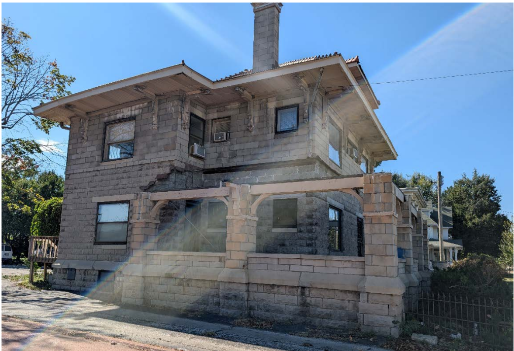
Photo 3 – Driveway Side Elevation; Facing West
