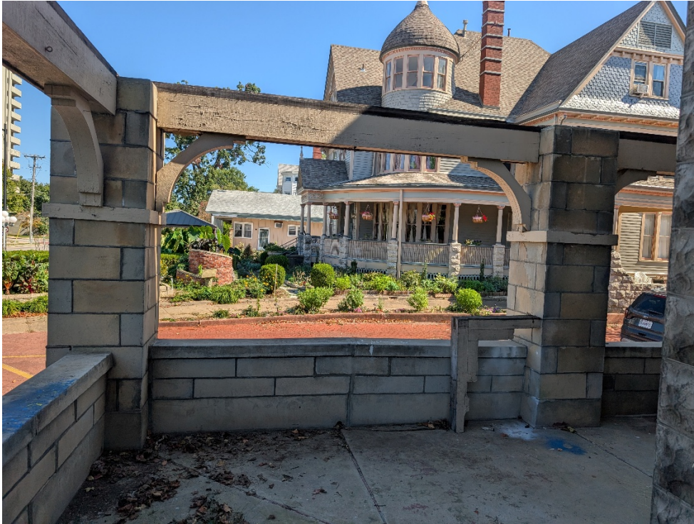
Photos 16-19 – Existing porch beams and support elements
