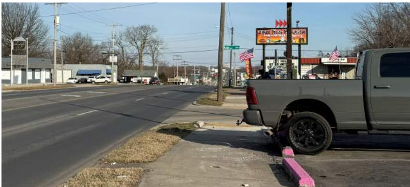
Parking Stops, Site Constraints, Non ADA Compliant.
