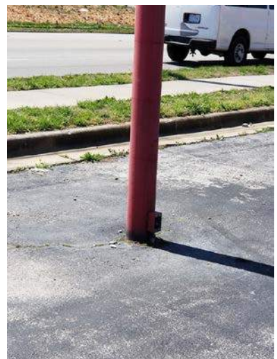
Figure 26 – Deteriorated signage w/ open junction box & exposed wires, 1200 block W Kearney St, north side
