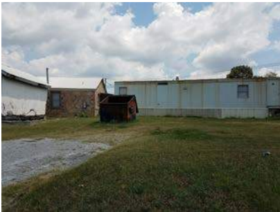
Figure 41 – 2300 block N Delaware Ave, east side
