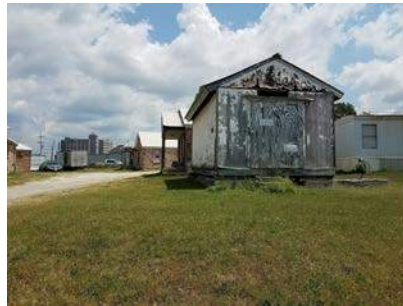
Figure 42 – 2300 block N Delaware Ave, east side
