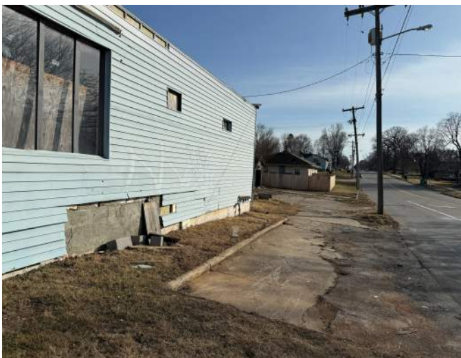
Located at 930 W Kearney, Building facade deteriorating. No sidewalk or curb. Non ADA Compliant.
