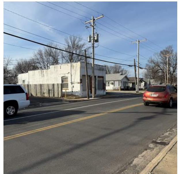
Located at 2407 N Grant, Building vacant and Boarded. Building appears to be in the ROW.
