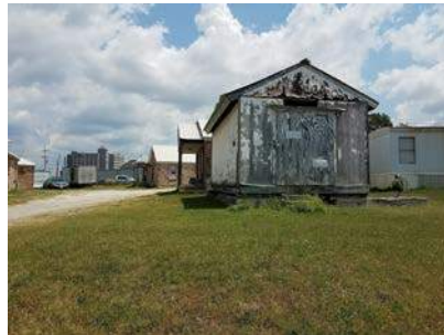
Figure 42 – 2300 block N Delaware Ave, east side
