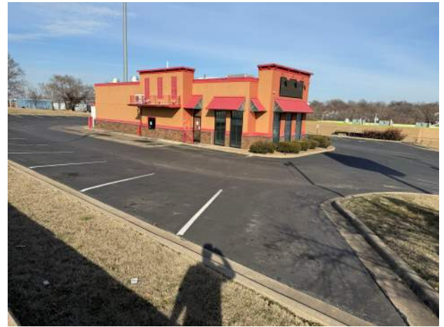
Located at 1421 W Kearney Building vacant.
