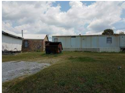
Figure 41 – 2300 block N Delaware Ave, east side
