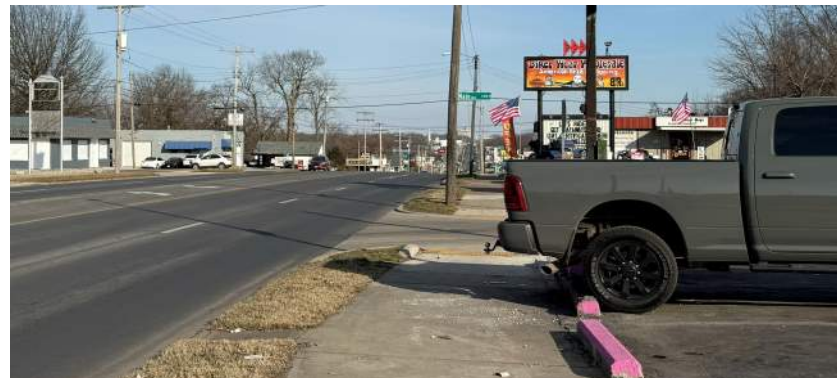
Parking Stops, Site Constraints, Non ADA Compliant.
