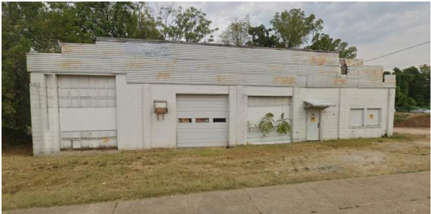
Located at 737 E Kearney. Buildings vacant and boarded. Inadequate site layout.
