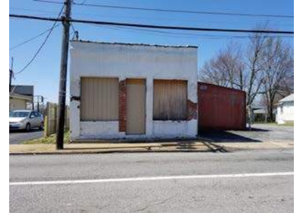
Figure 40 – 2400 block N Grant Ave, west side
