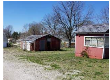
Figure 47 – 800 block W Kearney St, north side
