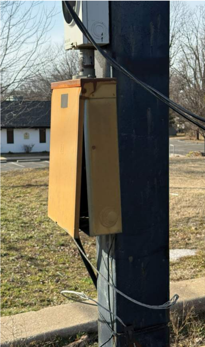
Located at 711 W Kearney, Signage has exposed electrical wiring and junction box. Deteriorated signage contributes to the blighted conditions of the corridor.
