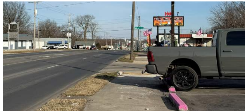
Parking Stops, Site Constraints, Non ADA Compliant.
