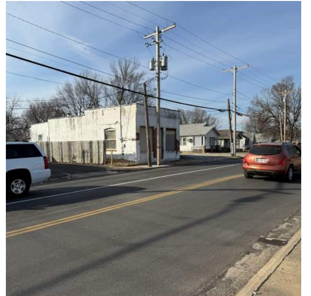
Located at 2407 N Grant, Building vacant and Boarded. Building appears to be in the ROW.
