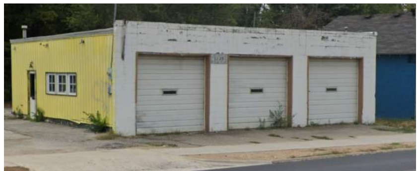
Located at 1326 E Kearney, Building deteriorating. Inadequate site layout.
