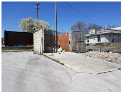
Figure 33 – 1300 block E Kearney St, north side
