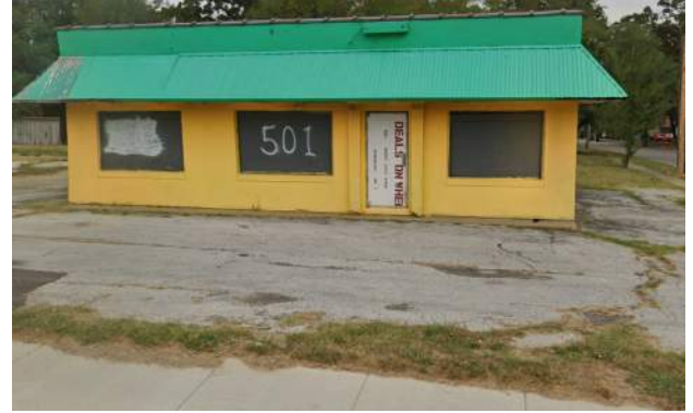
Located at 501 W Kearney. Buildings vacant and boarded. Inadequate site layout.
