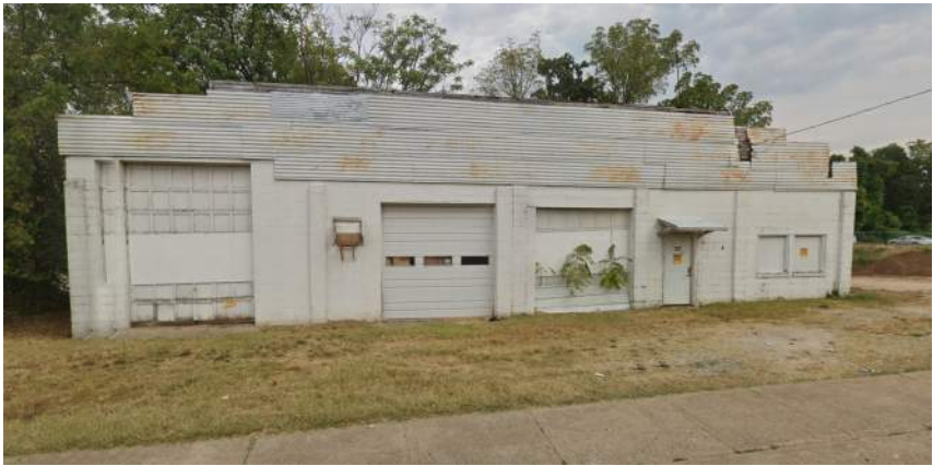
Located at 737 W Kearney. Buildings vacant and boarded. Inadequate site layout.
