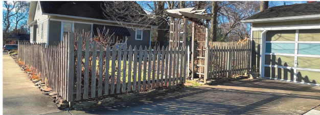
2 NORTH ENTRANCE FENCE & GATE AT DRIVEWAY
