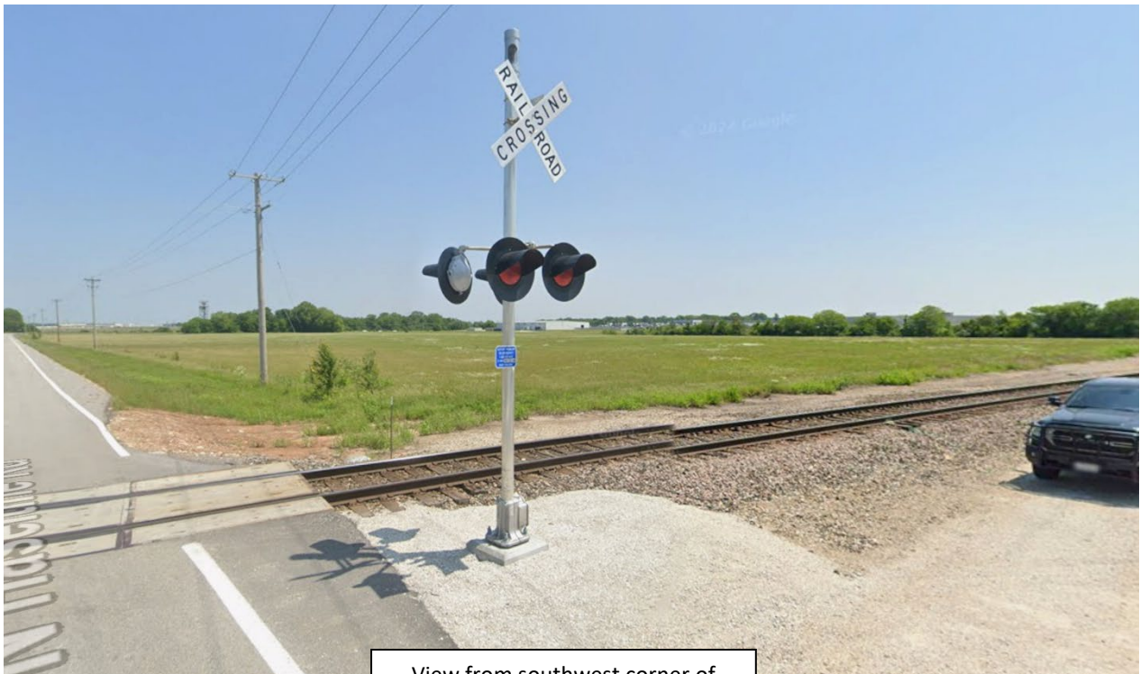
View from southwest corner of subject area
